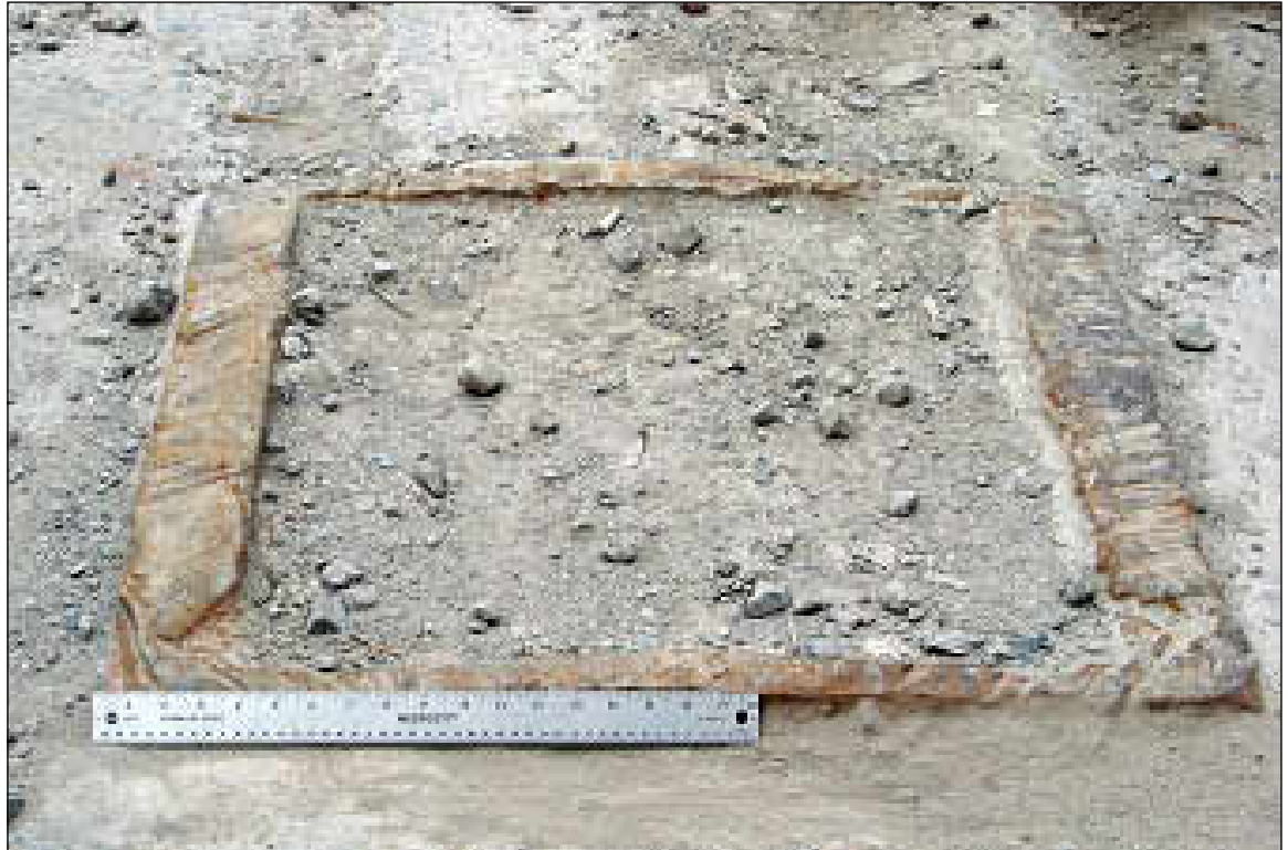
Bathtub area, detail view of box beam column footing
