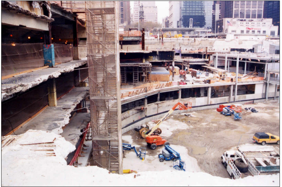
North slurry wall, view of remnants of 6 WTC
