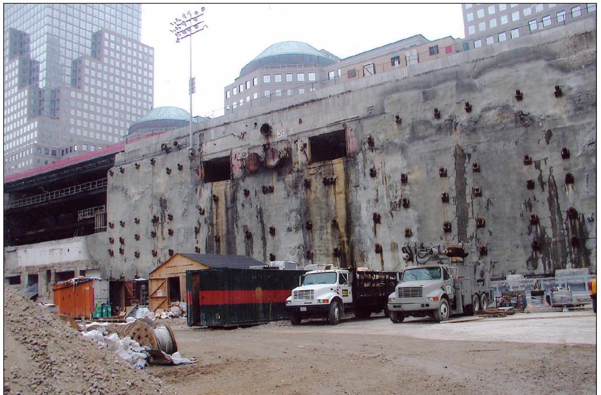
West slurry wall, view of vehicular entrance ramps and southern projection
