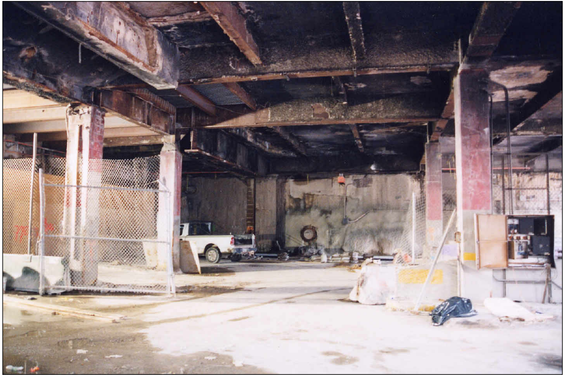
View of 6 WTC remnants, former area of below-grade parking
