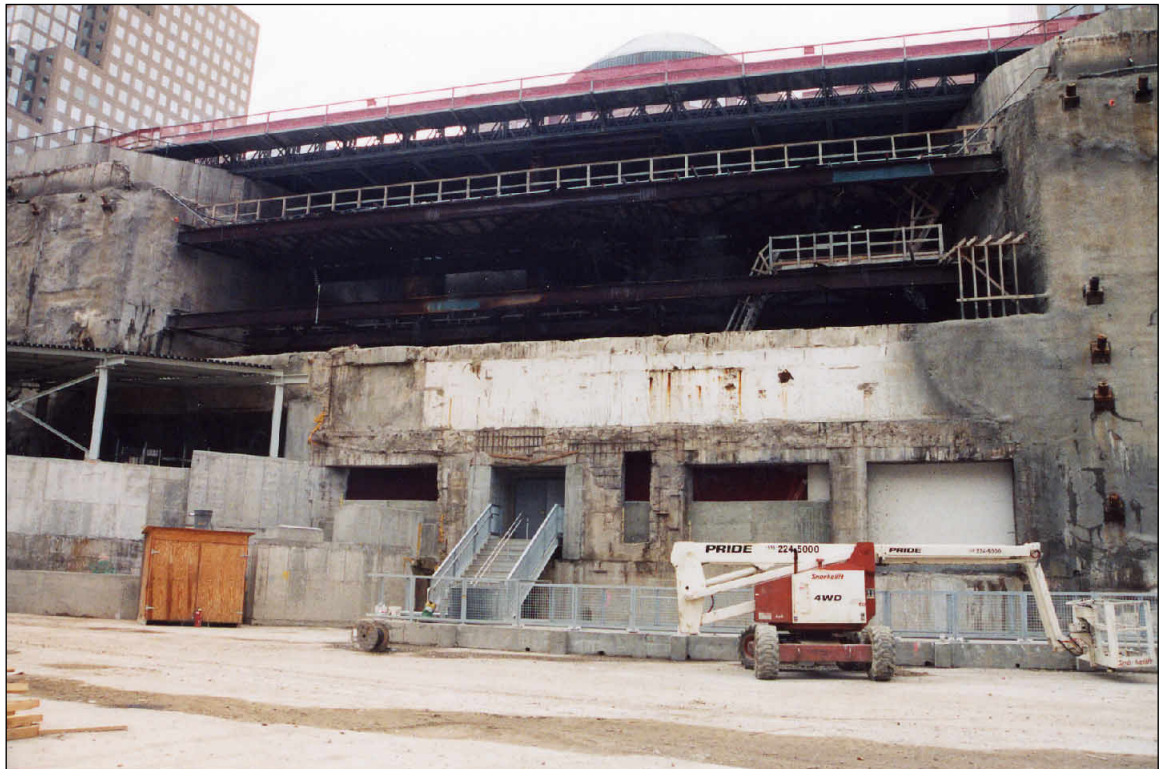
West slurry wall, view of southern projection and PATH tunnel access
