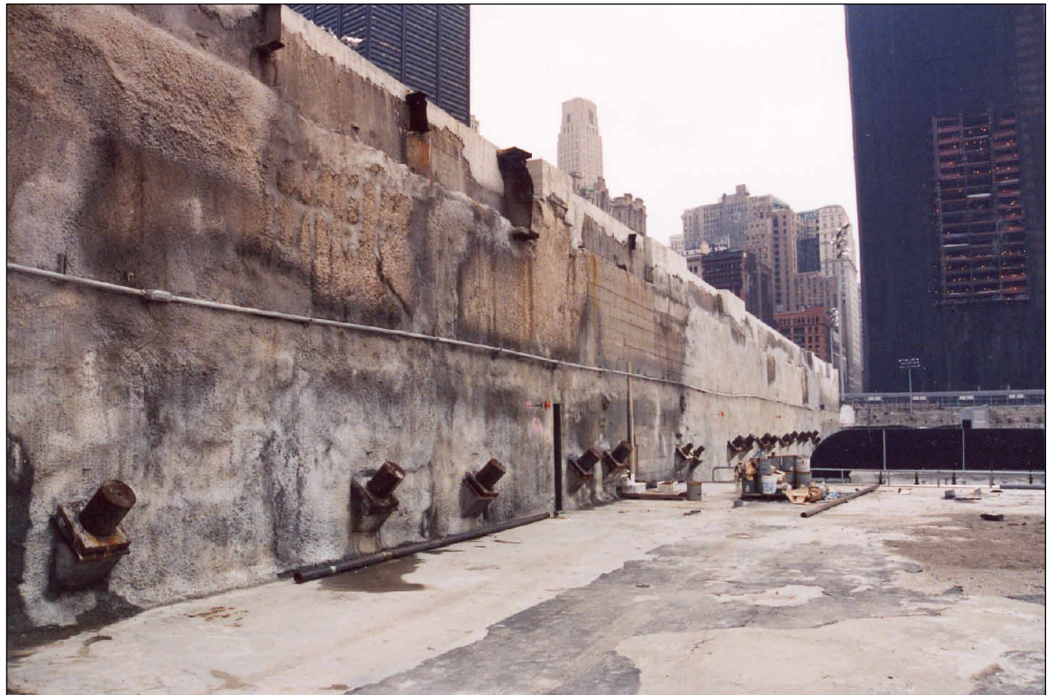
East slurry wall
