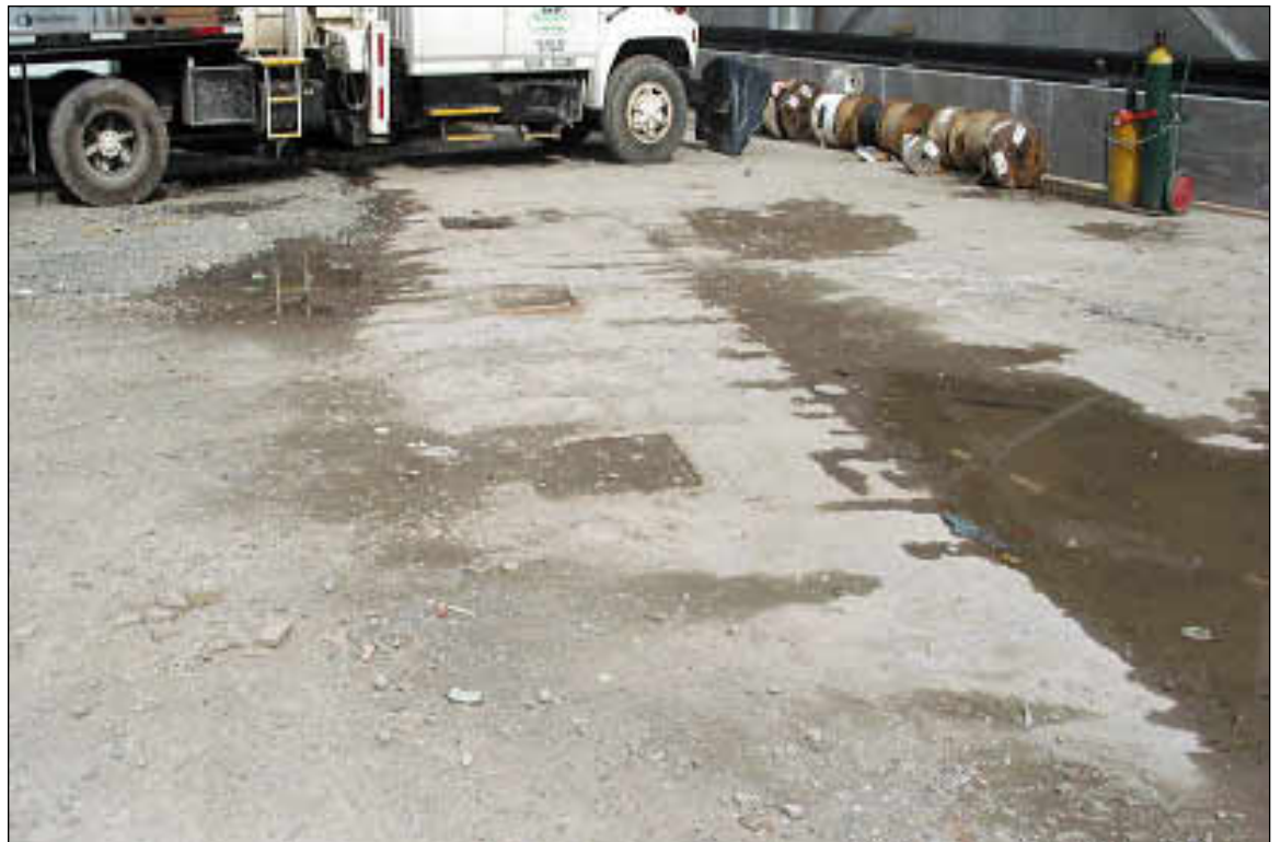
Bathtub area, box beam column footings
