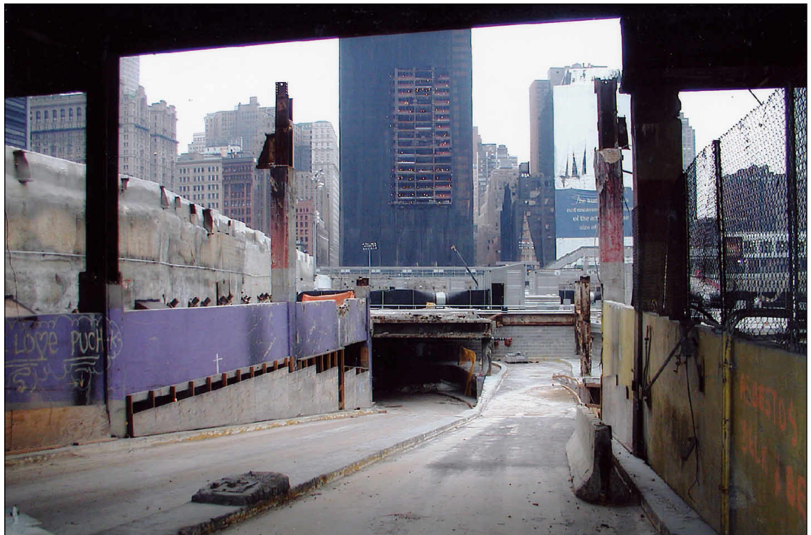
East slurry wall, view of vehicular access ramp
