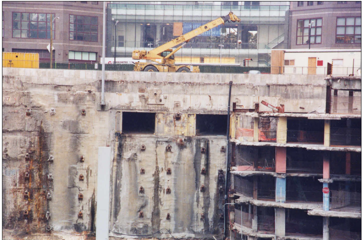
West slurry wall, north end
