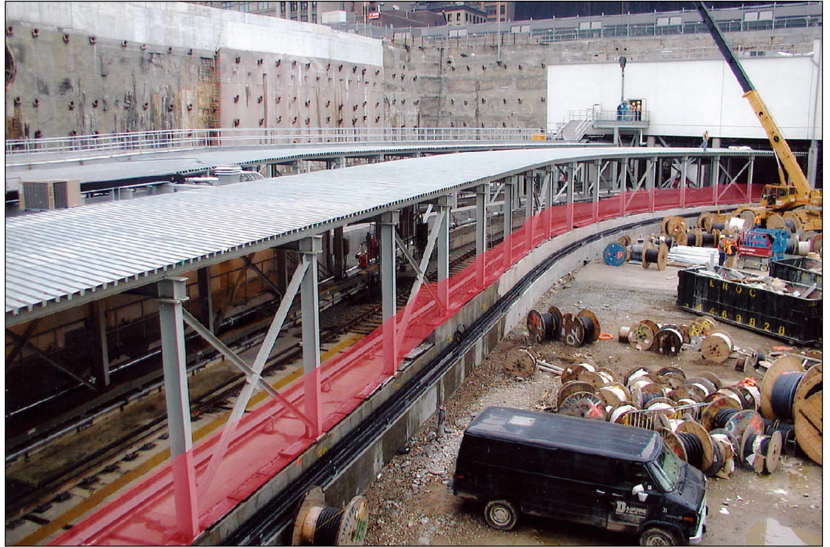
South and east slurry walls, view of new PATH tracks
