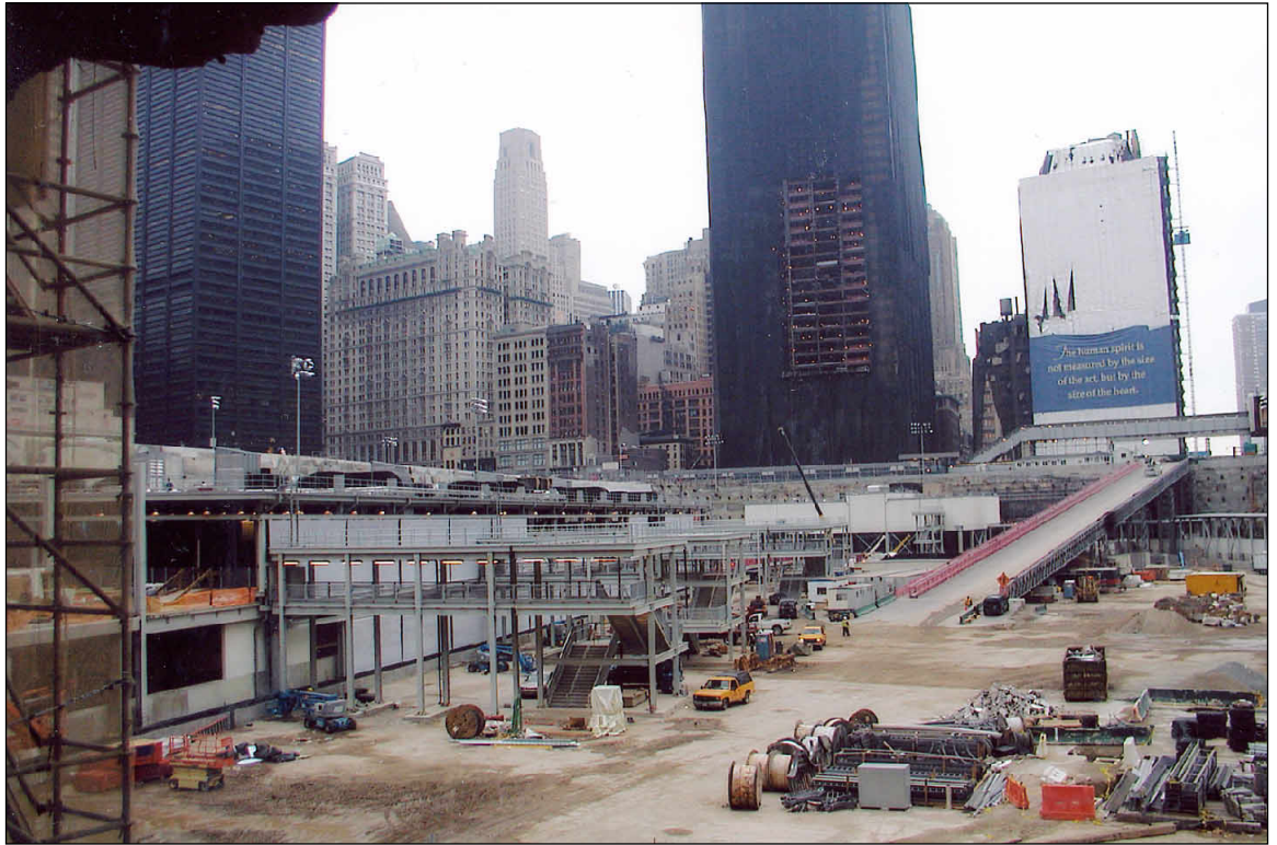
View of temporary WTC PATH station, adjacent to east slurry wall
