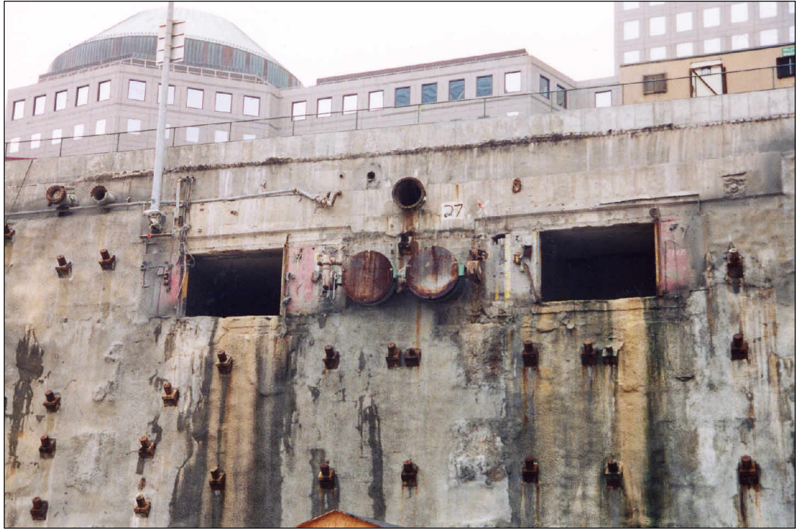
West slurry wall, detail view of vehicular entrance ramps
