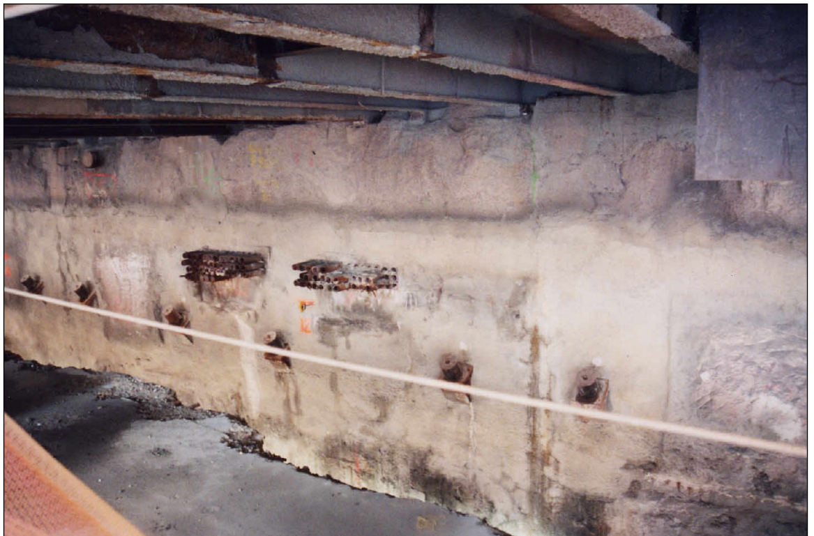
North slurry wall, view of temporary tiebacks
