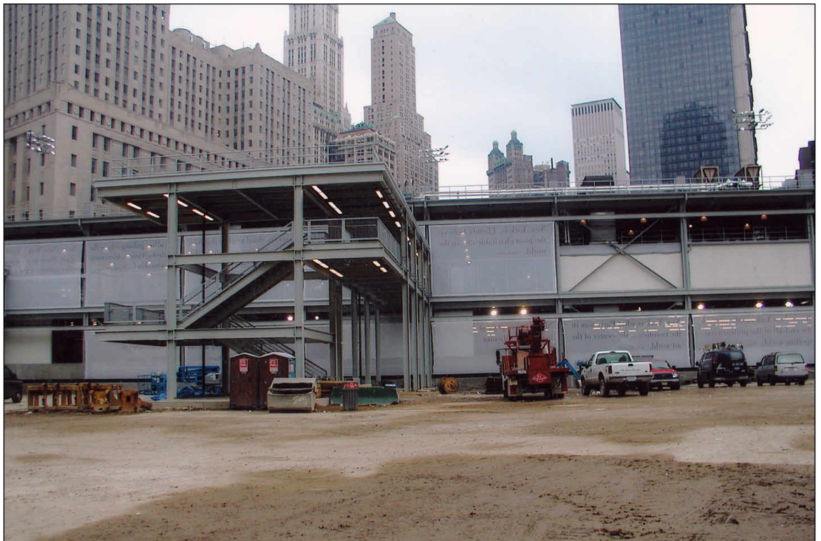
View of temporary WTC PATH station
