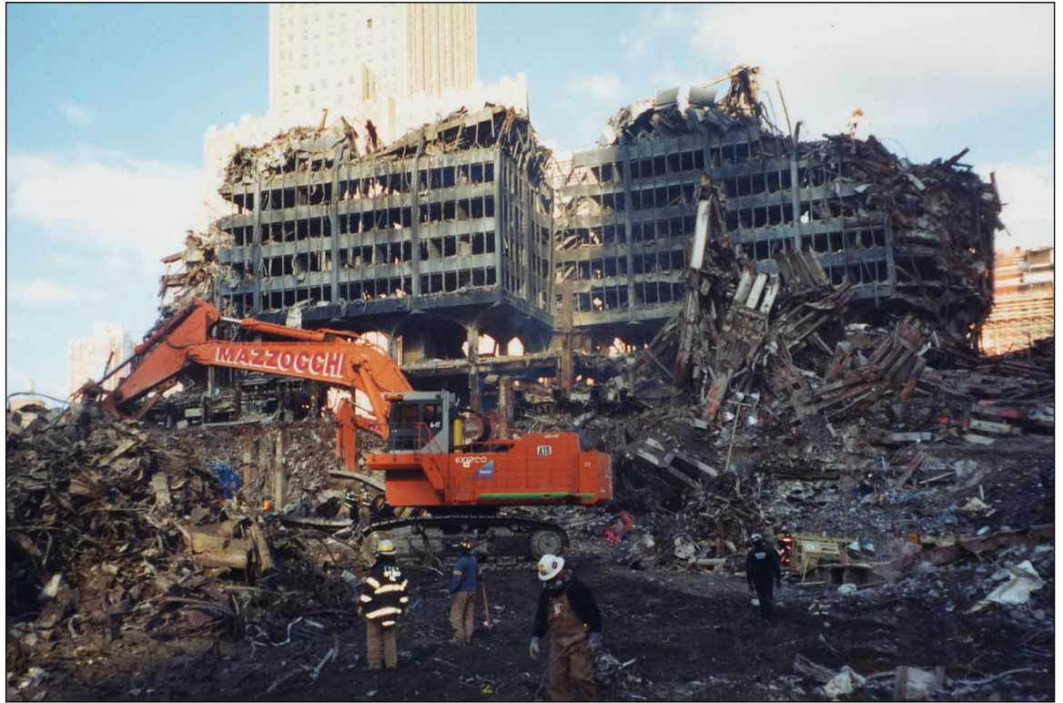
View of WTC Site as it appeared in December 2001 (Port Authority)
