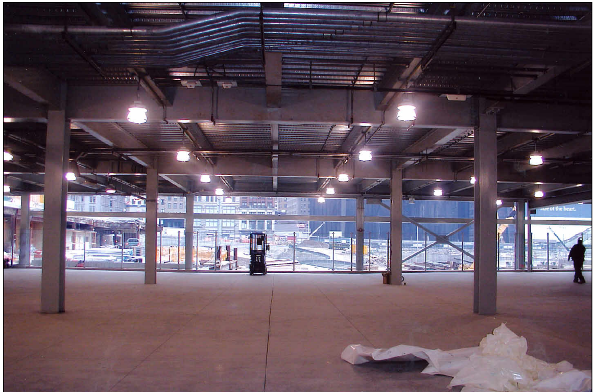
View of new temporary WTC PATH station concourse
