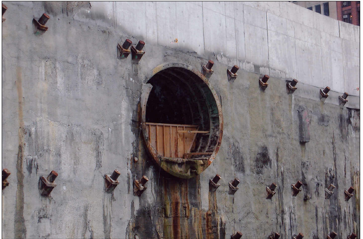
East slurry wall, view of Hudson Tube
