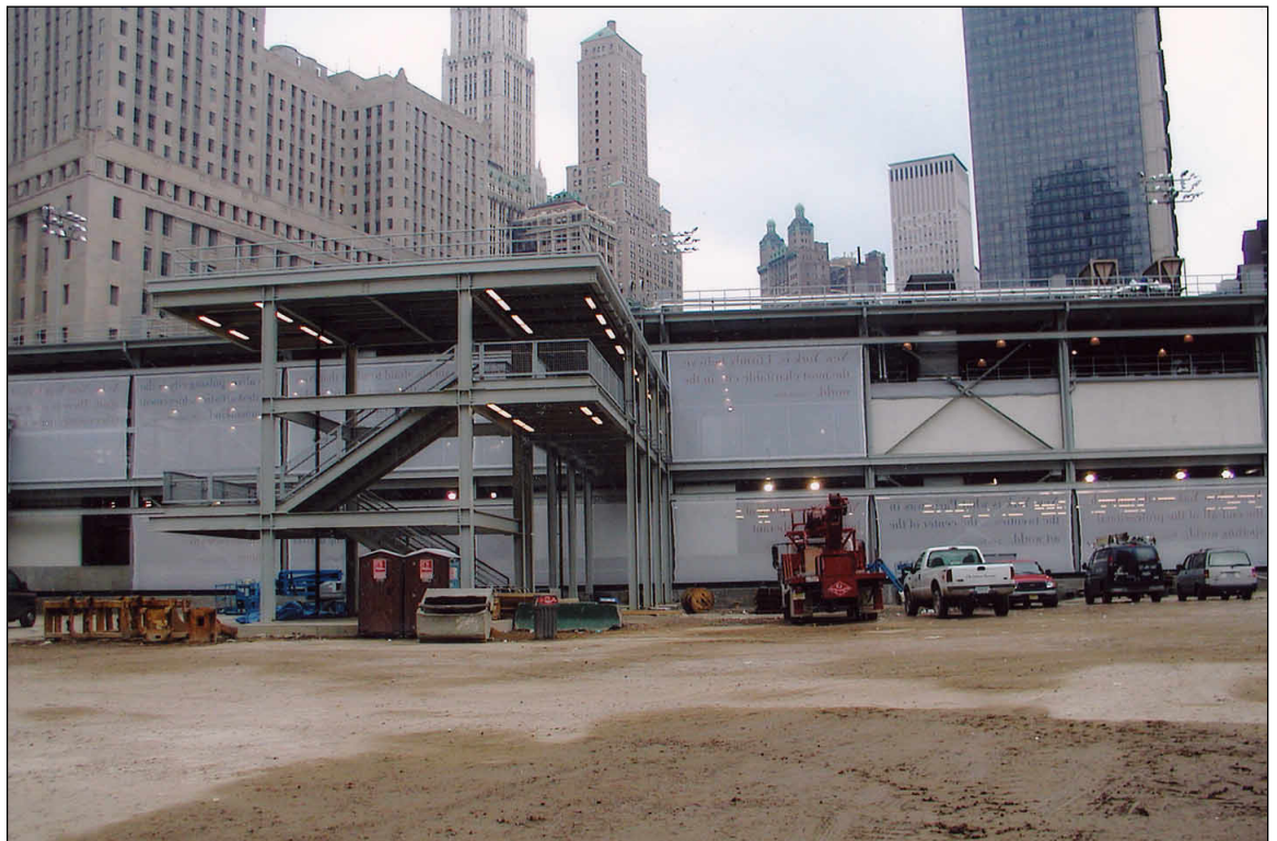
View of temporary WTC PATH station
