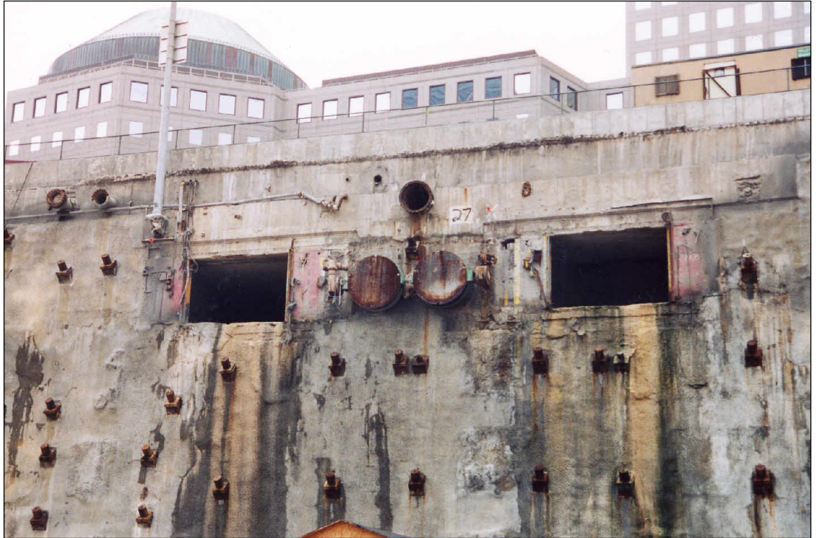
West slurry wall, detail view of vehicular entrance ramps and cooling water pipes
