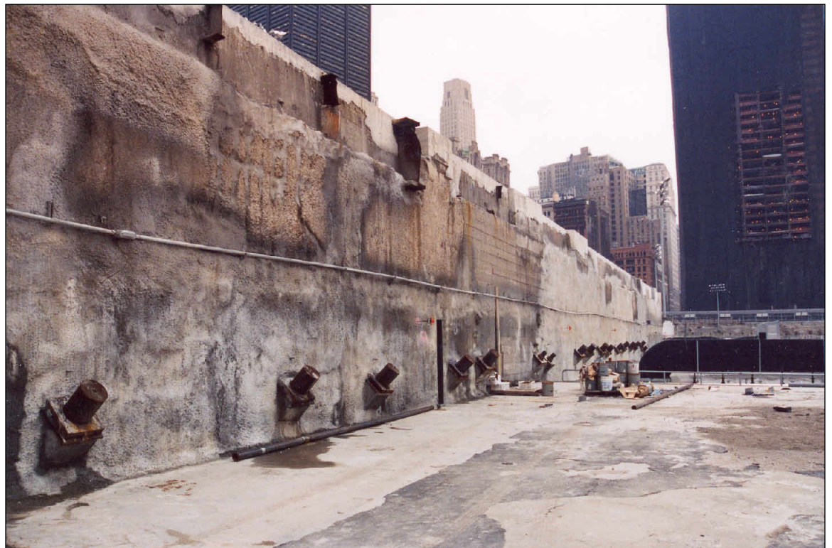
East slurry wall
