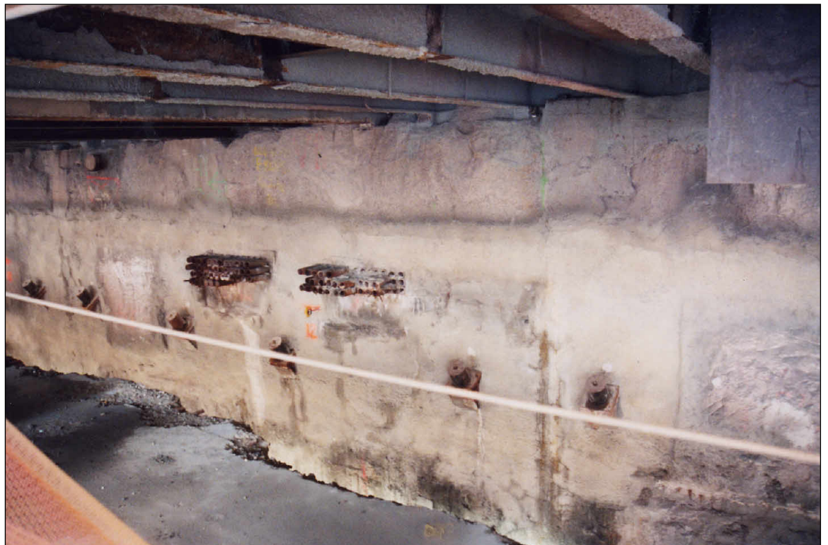
North slurry wall, view of temporary tieback caps
