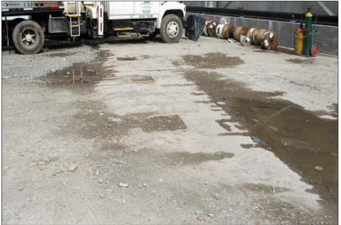
Bathtub area, truncated box beam column bases
