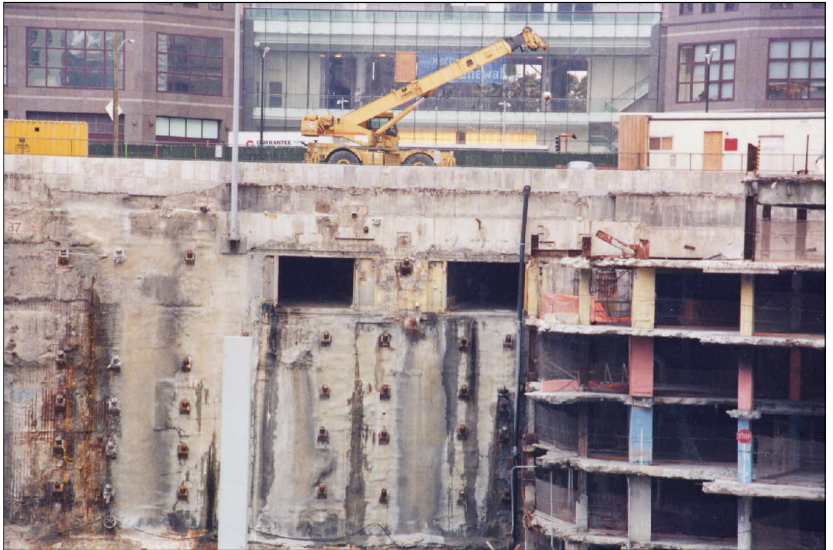
West slurry wall, north end
