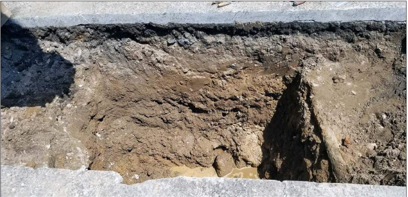
Facing north showing north wall of TP4. Note iron utility line along right side of trench, shallow, thick concrete pad on the left side of photo, mixed sandy fills, and water accumulating on trench floor at a depth of about 6 feet bgs **20**
