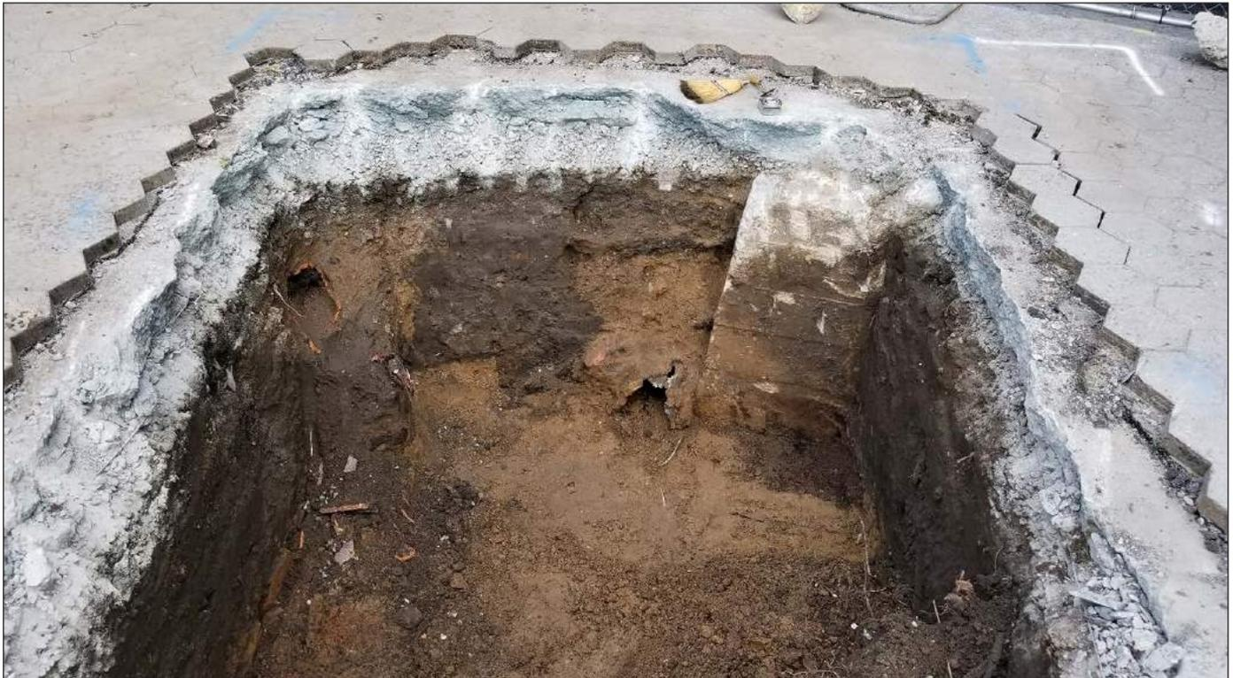
Facing west towards western wall of TP1. Note 6-foot-tall poured concrete pier in northwest corner of trench, disturbed soils, and fractured drainage line in southwest corner of trench. The trench floor is approximately 4 feet bgs in this photo 8
