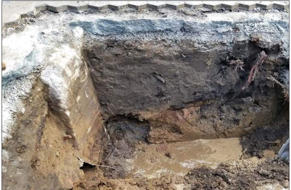
Facing north at the west end of TP1 showing the north wall profile and poured concrete pier to the left. Note that the floor of the trench is filling with water at a depth of about 6 feet bgs **9**
