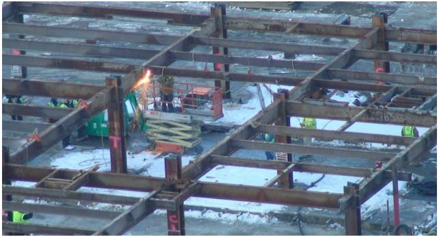
Scissor Lift – used at 130 Liberty Street to hoist welders up to the steel beams.
