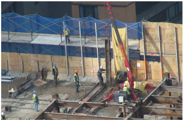
**Spyder Crane** – the small size and maneuverability of these mini-cranes allow them to be used where other cranes cannot go. On the 130 Liberty Street project the mini-cranes are used to access the interior of the building, hold steel in place, and lower steel onto the deck.
