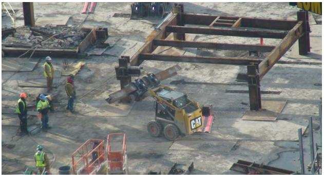
**Skid Steer Loader** - used to move building materials such as steel on the deck of 130 Liberty Street. Their small size and maneuverability allows them to operate in tight spaces.
