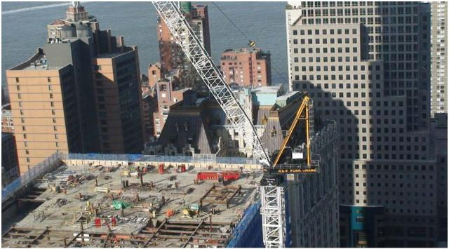
**Tower Crane** – a common fixture at any major construction site. They often rise hundreds of feet into the air, and can reach out just as far. The construction crew uses the tower crane to lift steel, concrete, large tools like acetylene torches and generators, and a wide variety of other building materials. On the 130 Liberty Street project the tower crane is used to lower large containers from the working deck to the ground. (As of January 29, 2010)
