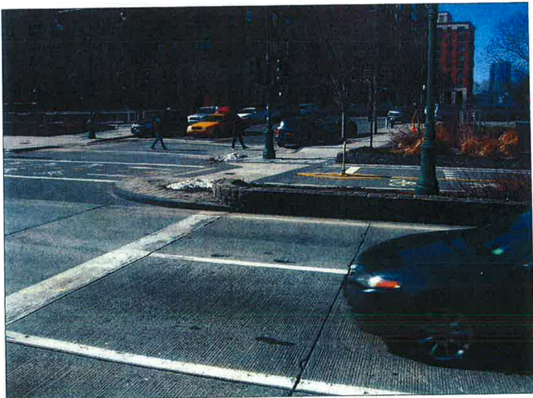
Plate 6. View to southeast from West St. median.
