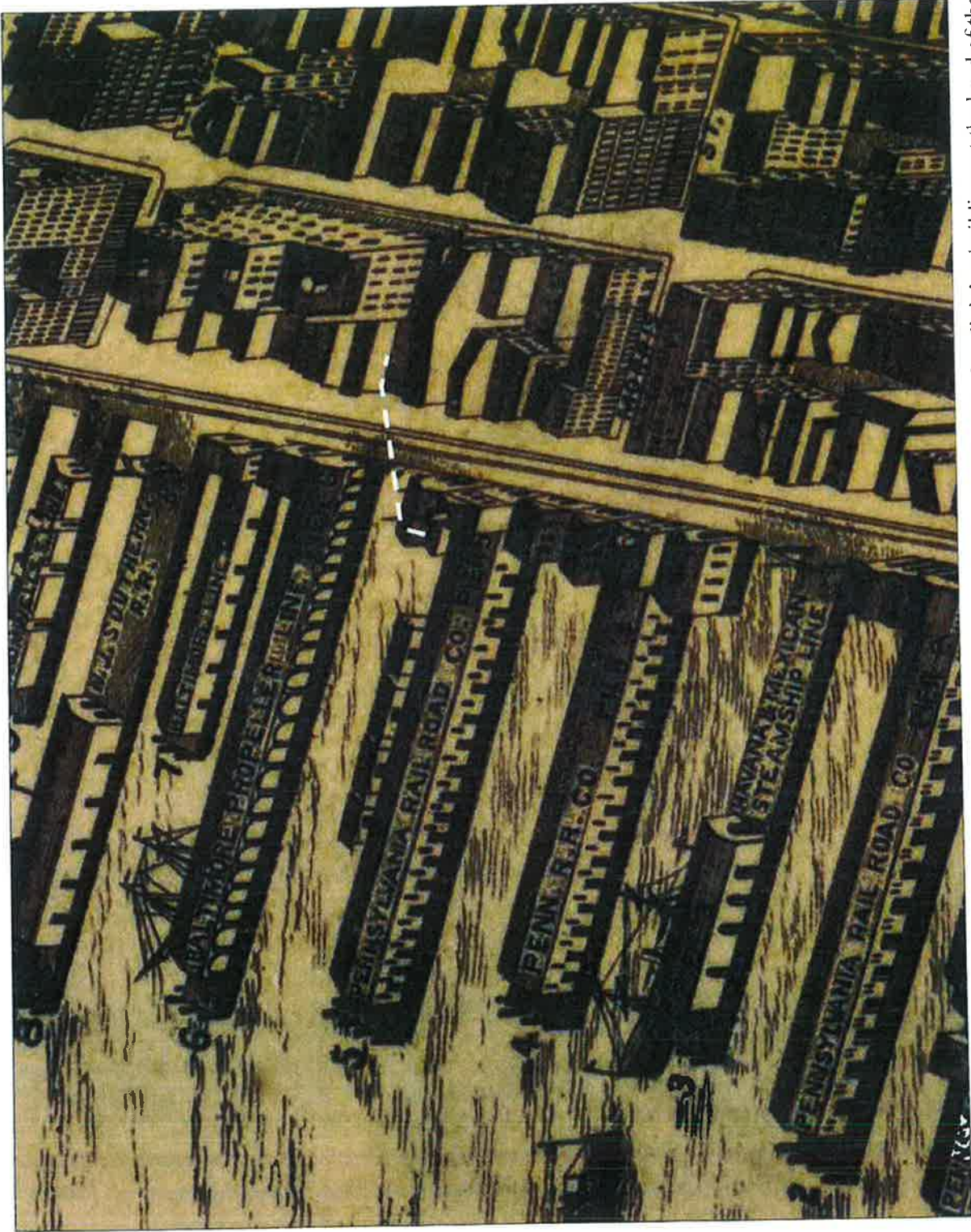
Figure 12. Detail from the Will L. Taylor bird's-eye view of New York in 1879. The six adjoining buildings at the head of the Pennsylvania Railroad piers (Piers 4 and 5) were on pilings, occupying space between West Street and the new (1871) bulkhead line. The project area is shown with dashed white line.
