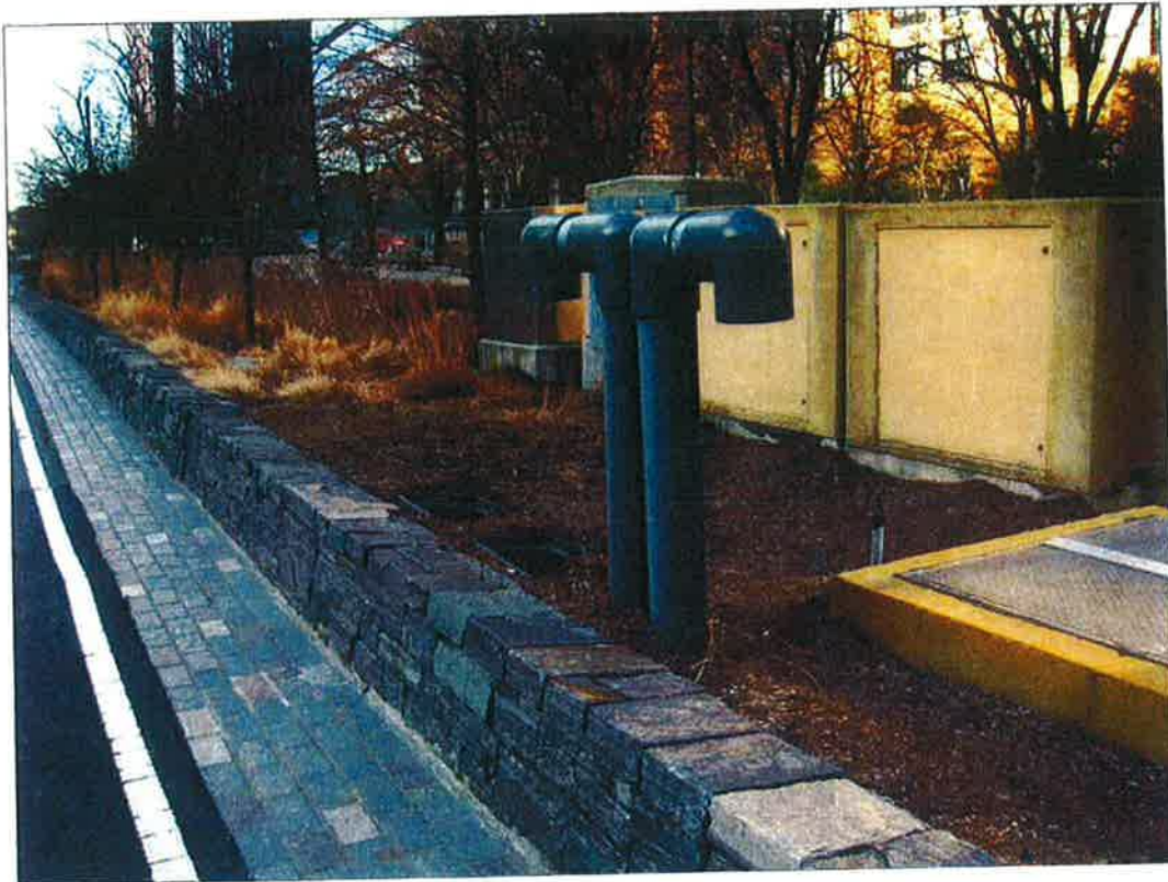
Plate 9. View of landscaped island within esplanade with utilities.
